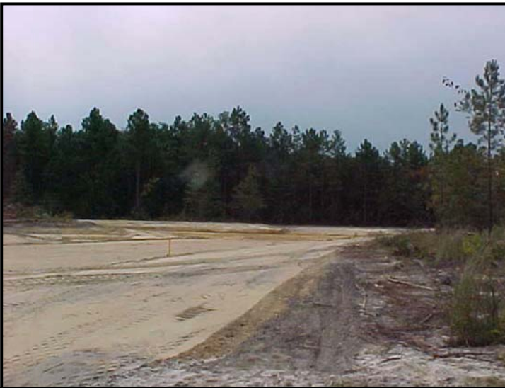
Looking at site from Longreen Parkway
