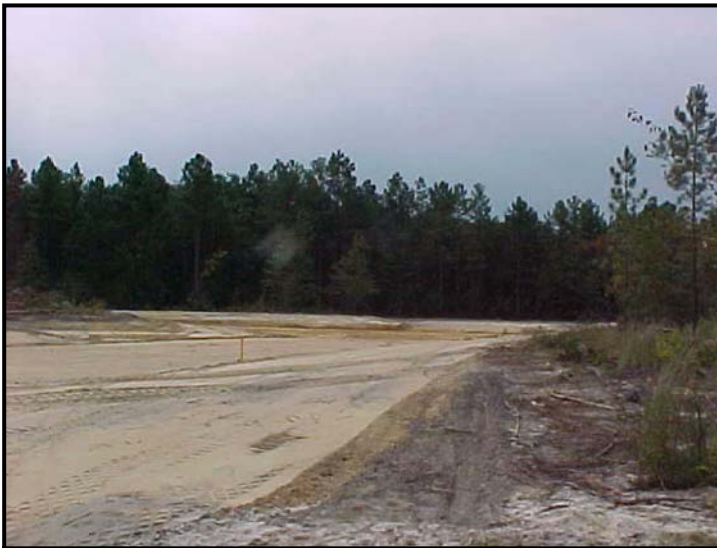
Looking at site from Longreen Parkway
